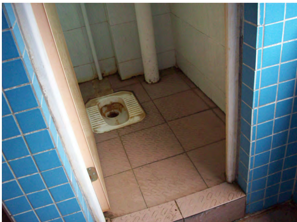
Image 9: Dormitory bathroom, picture from 2008 report
