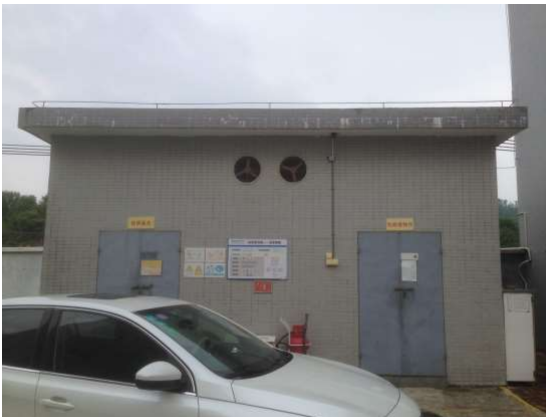
Storage shed for hazardous chemicals and chemical waste
