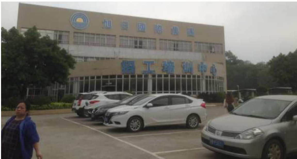
(Training center for new hires, the first floor is the recruitment lobby, second floor is where the training classroom is located)
