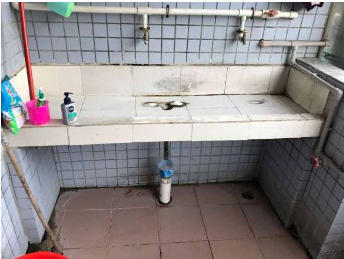
Sink area of the dormitory
