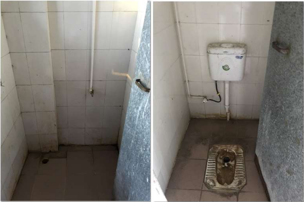
Restroom of the dormitory
