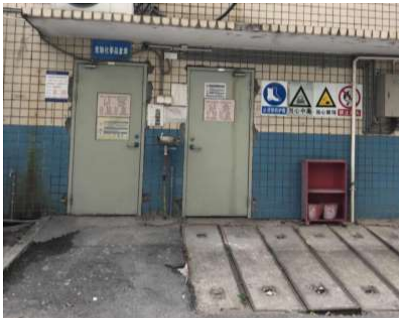
Hazardous chemicals storage unit
