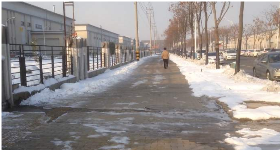
Factory's wastewater flowing overflowing onto the sidewalk
