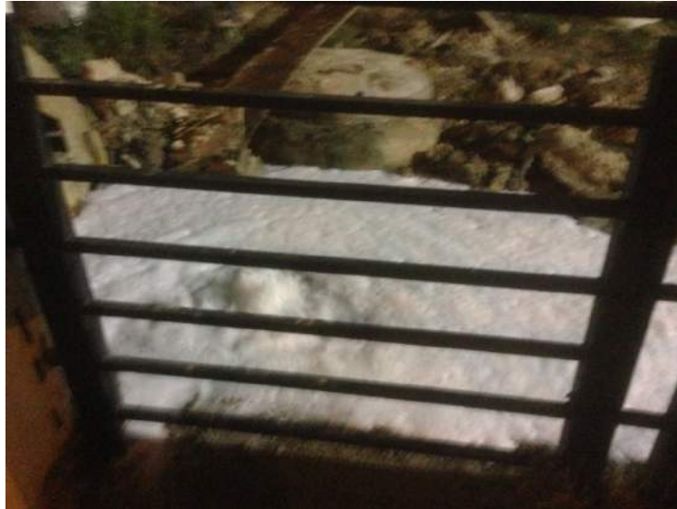
Factory wastewater bubbling up from underground sewer pipes. A water sample here was taken for testing.
