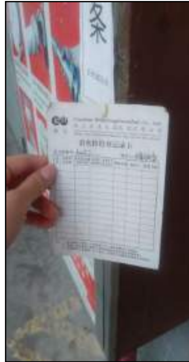
Fire extinguishers have no record of past inspection
