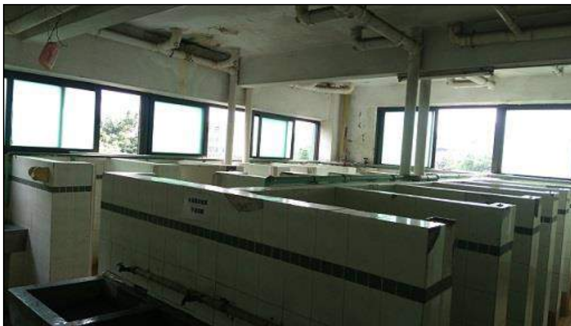
Bathrooms in the dormitory
