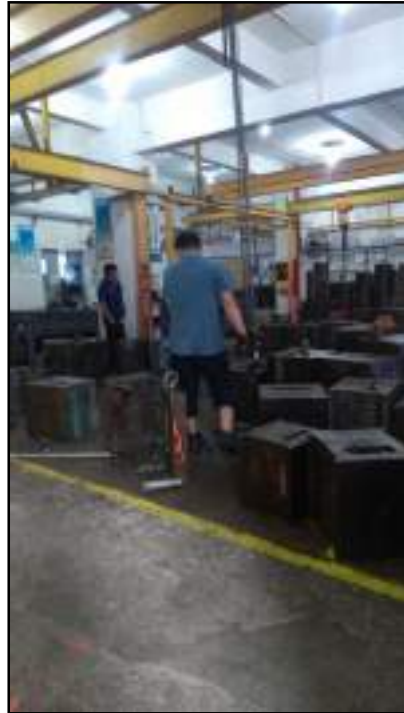
Workers working with molds do not have safety helmets
