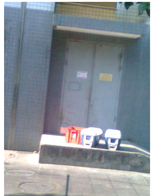
The emergency exit door is closed and debris piled up and block the exit
